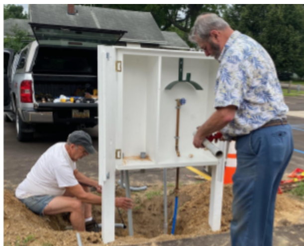
Jerry Dundon and Bert Ogden work on the parking lot: Two separate boxes, per code, left box for electricity plus internet, right for water. Any volunteers for landscaping?
